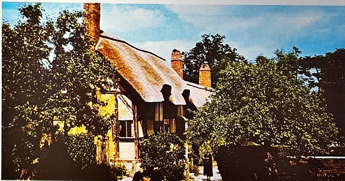
Anne Hathaway's Cottage, Shuttery
